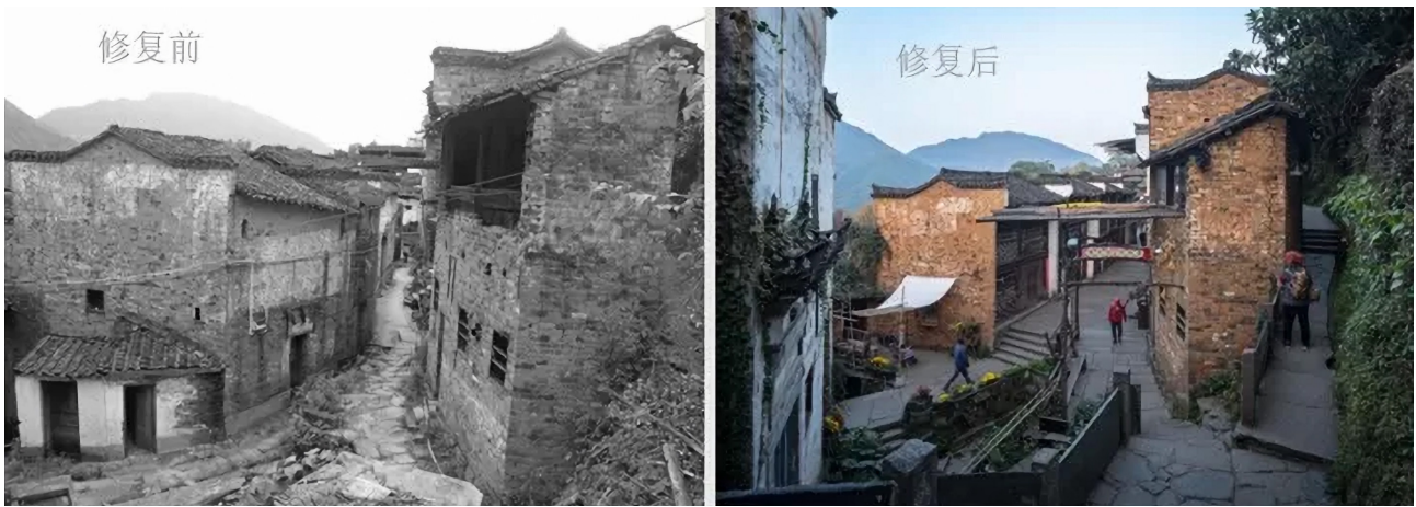
Figure 11. Renovation and Transformation of a Village 7.
