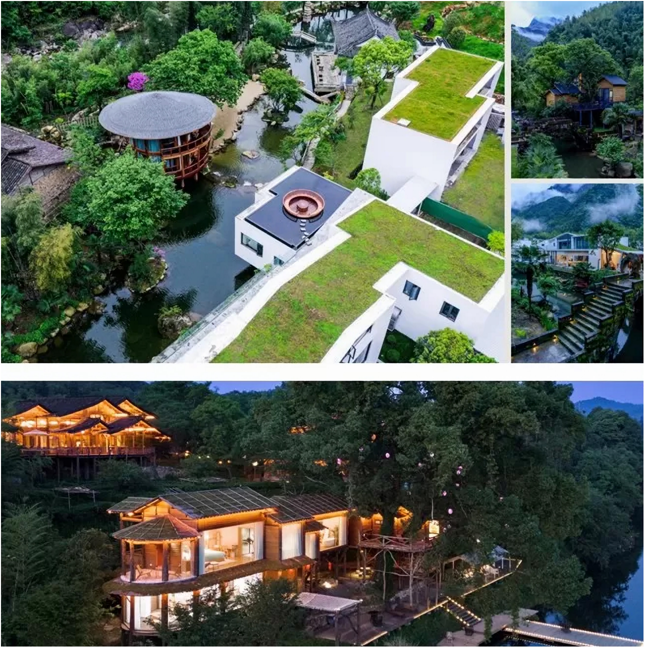
Figure 12. Renovation and Transformation of a Village 8.
