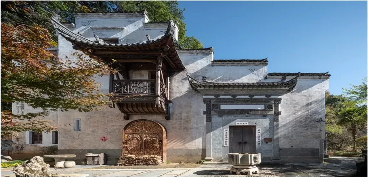
Figure 9. Renovation and Transformation of a Village 5.
