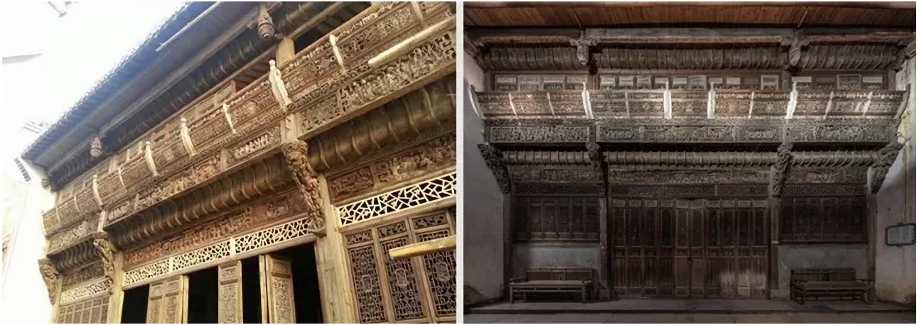
Figure 9. Renovation and Transformation of a Village 5.
